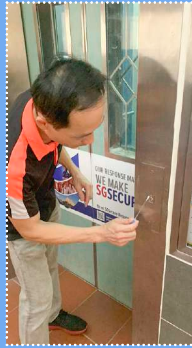
Applying a self-disinfecting coating (SDST) to lift buttons kills germs and prevents them from breeding. After application, the ATP reading of bacteria count drops to zero
