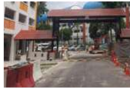
Linkway at Blk 863 Yishun Ave 4 to Naval Base Primary School
