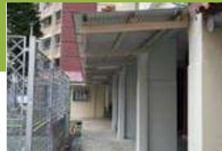
Awnings at Blk 250, 259 and 260 Yishun St 22/Ave 9
