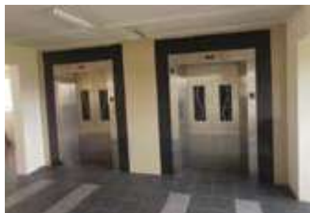
Upgrading of lift lobbies at Blk 926, 927, 928, 930, 931, 932 and 935 Yishun Central 1
