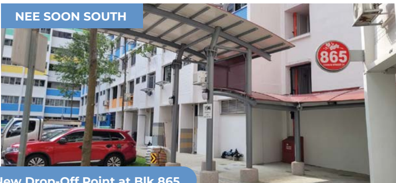
New Drop-Off Point at Blk 865
