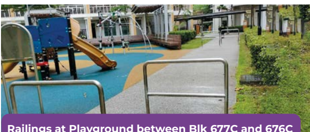
Railings at Playground between Blk 677C and 676C
